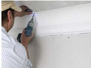
Fix article on metal structure using screws.
