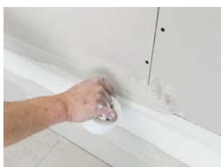
After applying second layer, lay mesh tape.
