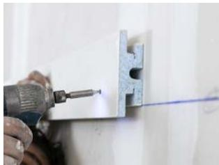
Fix article using screws.
