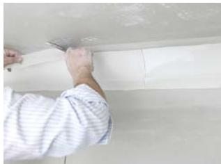
After applying second layer, lay mesh tape.
