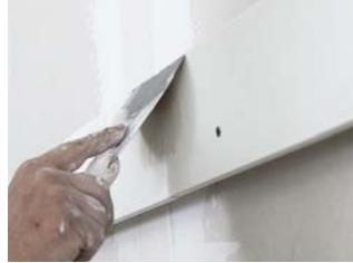
Plaster along joint between the two profiles.
