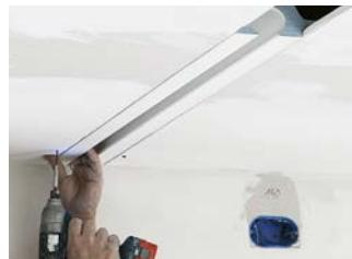
Fix article onto false ceiling using screws.
