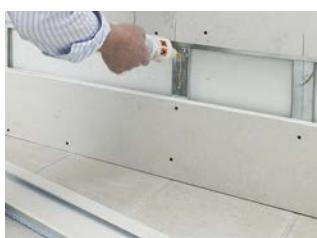
Apply adhesive on the metal structure.
