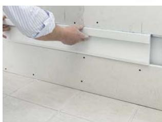
Fix article on metal structure using screws.
